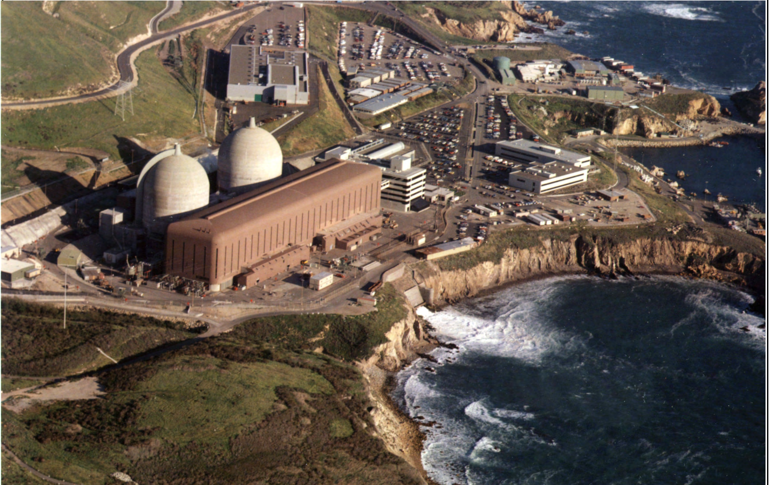
Diablo Canyon Nuclear Power Plant in California.
