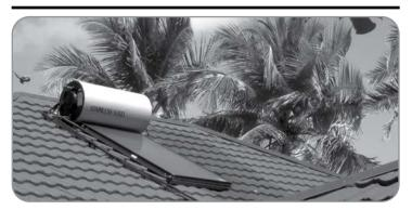
The heated fluid then goes to a storage tank where it heats water. The hot water may then be piped to a faucet or showerhead. Most solar water heaters that operate in winter use a heat transfer fluid, similar to antifreeze, that will not freeze when the weather turns cold.
