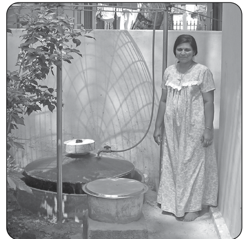
Photo courtesy of Ashden Awards for Sustainable Energy This woman in India has a biogas tank in her backyard. Biogas provides her home with energy for cooking and lighting.
