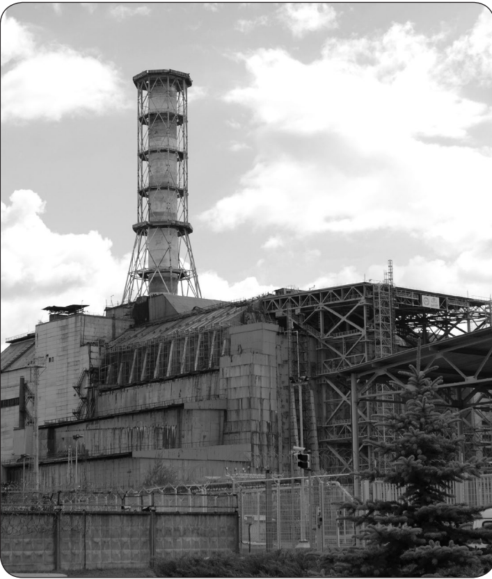
The damaged reactor number four of Chernobyl Nuclear Power Plant
